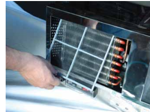
Step 3-4. Replace the cleaned AIR FILTER
